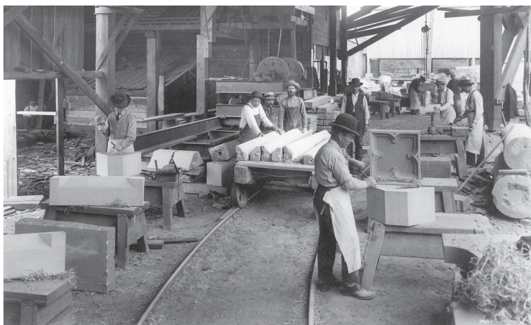
Work shed of Hercules Sandstone Co. Quarry No. 1, Tenino, where workmen shaped blocks of sandstone, 1909. Andrew Wilson, lead stonecutter, is in foreground. (University of Washington Special Collections, Neg. No. A. Curtis 14652).
