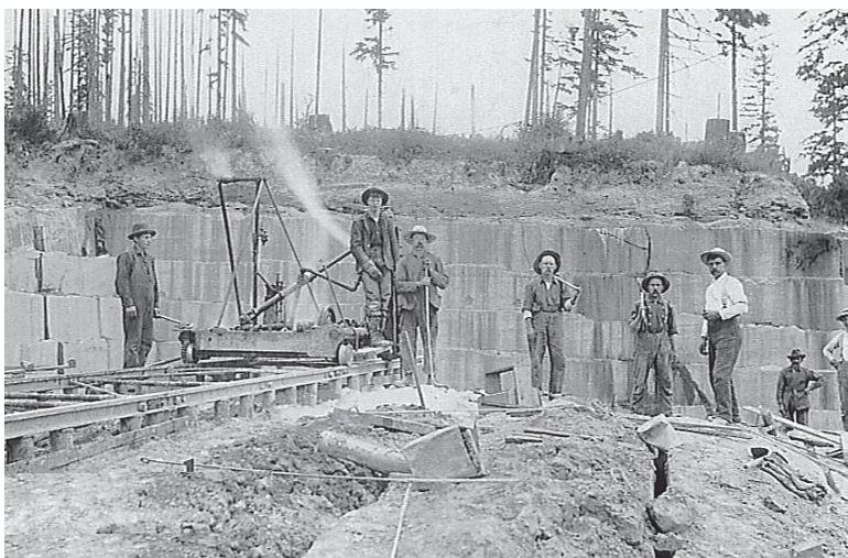
Stone cutting channeler at Hercules Sandstone Co. Quarry No. 1, about 1905. This was a steam-powered channeler. The steam came by hose from a stationery boiler. (Marenakos Rock Center Collection)
